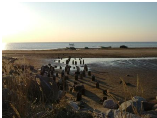
Figure 6.5. Pylons of the Southern cargo jetty of Ainazi port
