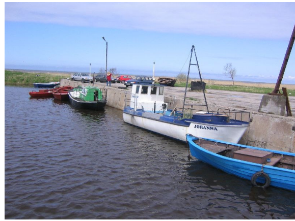
Figure 6.10. The Northern berth of Treimani port
