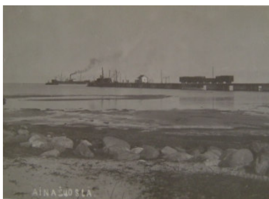
Figure 6.1. The Southern cargo jetty of Ainazi port before the First World War Source: Ainazi City Council
